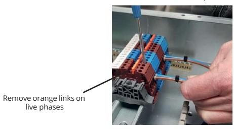
Undo the terminals and remove the power feed wires from the terminals. Route these back down the trunking to become your "live feed" for the associated DIN lighting module.
