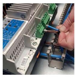
Then wire from the DIN module outputs to the terminal blocks (usually 4 outputs using correct wire).
